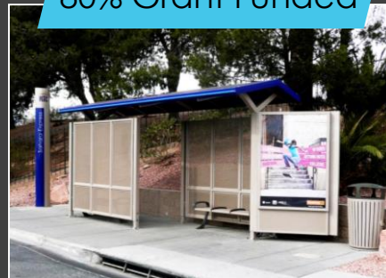
Bus Shelters & Safety Enhancements $7.6 Million
